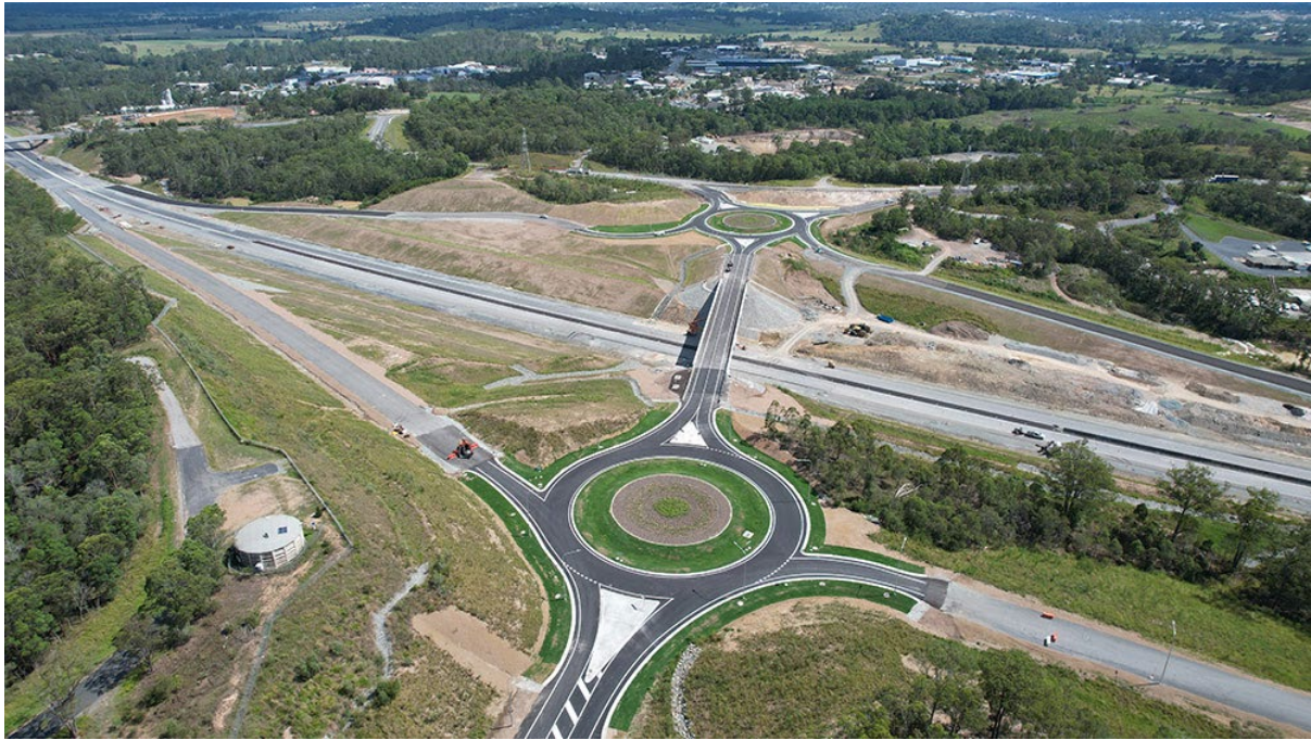
Figure 3: Flood Interchange aerial view of completed work as at December 2022
