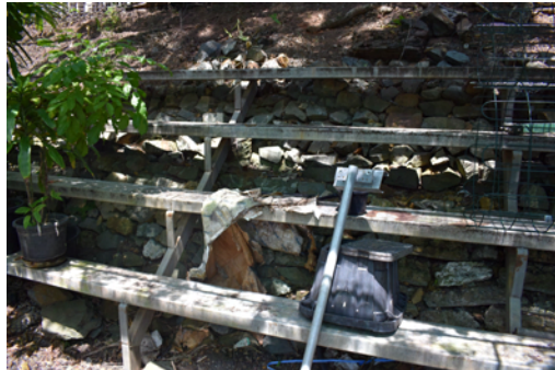
The basalt rubble wall, behind the tiered pot plant stand, with white painted stones which likely date from the original ca. 1919 rockery. There are pieces of old concrete slab used in the lower part of the retaining wall.
