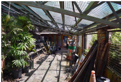
Interior of the fernery facing the storage shed.
