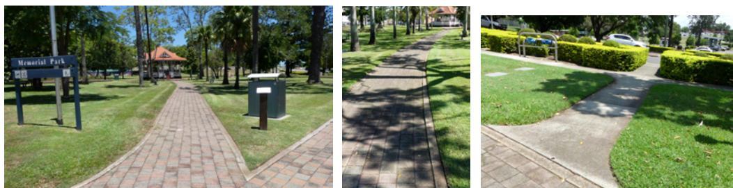
The avenue pathways have concrete unit pavers between concrete edges
