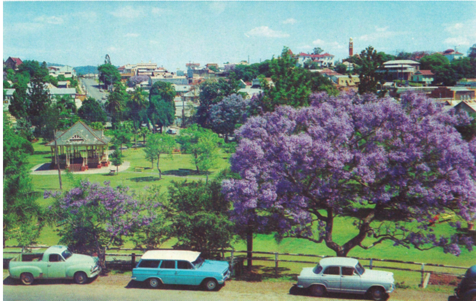
Very early 1960s view across Young Street towards Reef and Monkland Streets. The original fibre cement bandstand roofing can be seen in deteriorating condition and the bandstand itself has a different colour scheme to today. Stair entrances are now on both sides of bandstand. Also of note is the original concrete surround. The east path (avenue C) is not yet paved.
