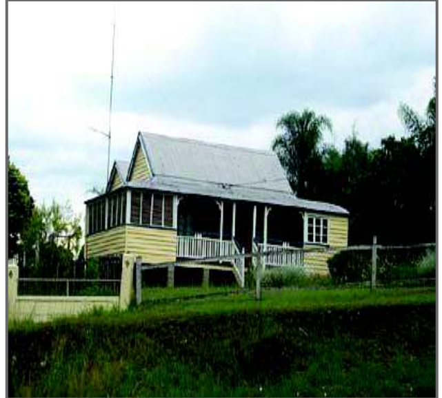
Photo sourced from Mark Baker Town Planning Consultants Pty Ltd in association with Ivan Mc Donald Architects
