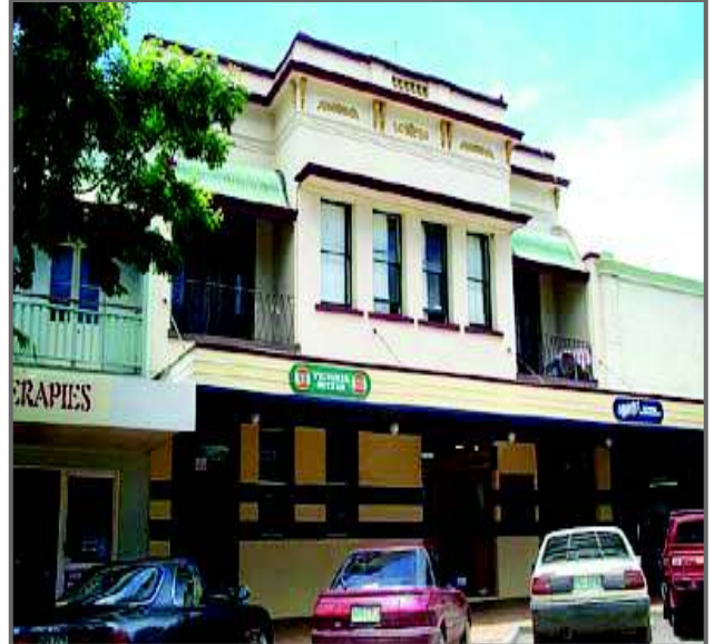
Photo sourced from Mark Baker Town Planning Consultants Pty Ltd in association with Ivan Mc Donald Architects
