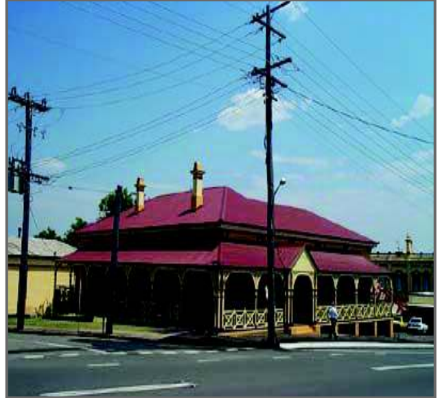
Photo sourced from Mark Baker Town Planning Consultants Pty Ltd in association with Ivan Mc Donald Architects
