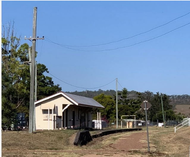
Goomeri Railway Station (former), 2020
