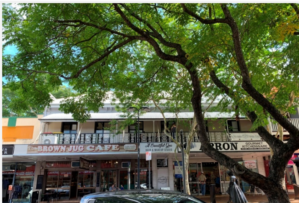
Walker's Building (former), 2019.
