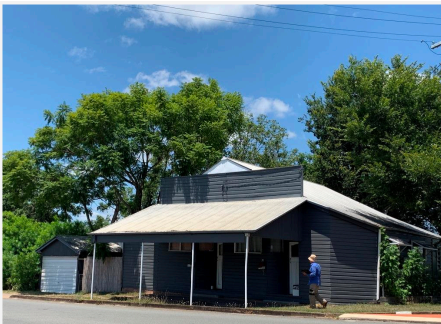
Commercial (former): 15 Graham Street, Gympie, 2019.
