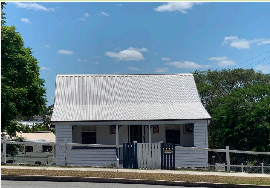
Residence: 10 Graham Street, Gympie, 2019.
