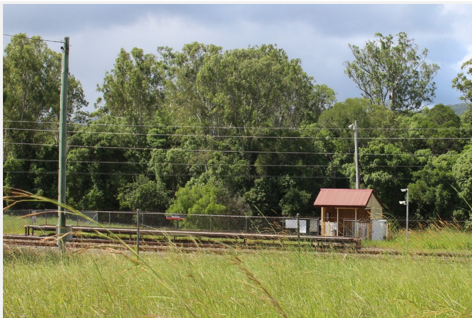
Traveston Railway Station, 2020.
