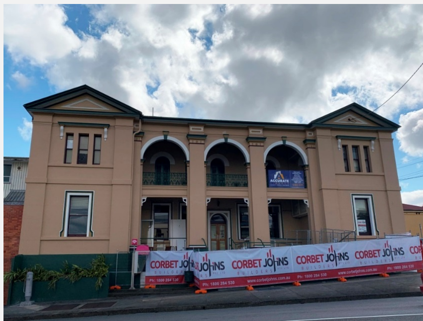
Gympie Post Office (former), 2019.
