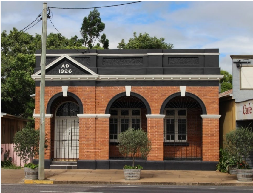
Queensland National Bank, Goomeri (former), 2020
