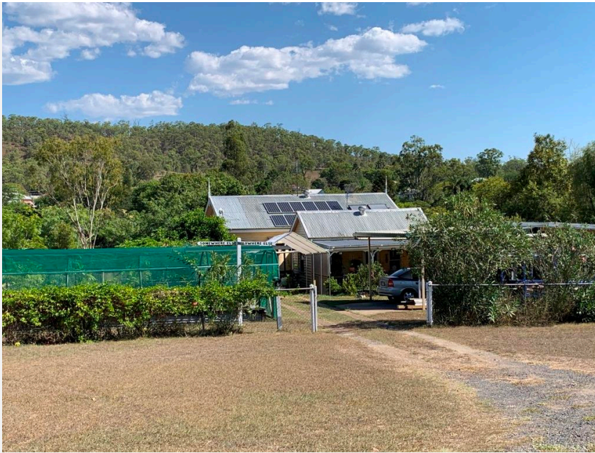
Kilkivan Station Master's Residence (former), 2019.
