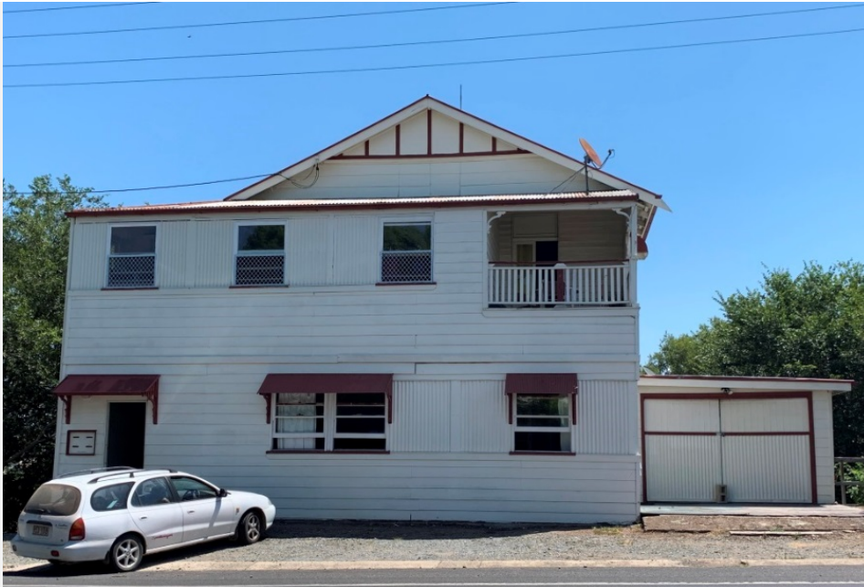
Gympie Fire Station (former), 2019.
