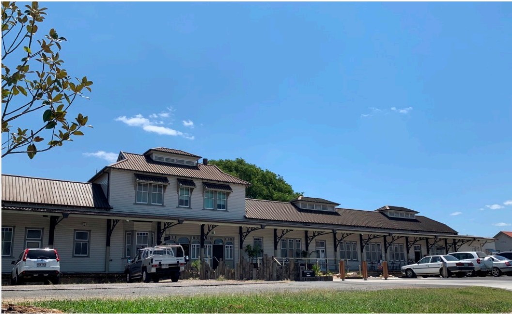
Gympie Railway Station Platform Complex, 2019.
