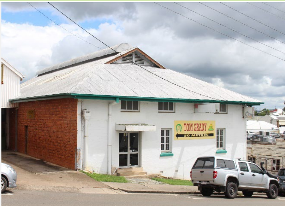
Southern Electric Authority Electricity Supply Building (former), 2020
