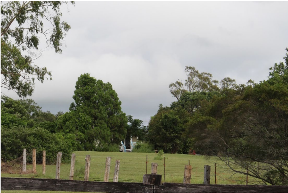
Residence: 33 Mudlo Road, Kilkivan, 2020
