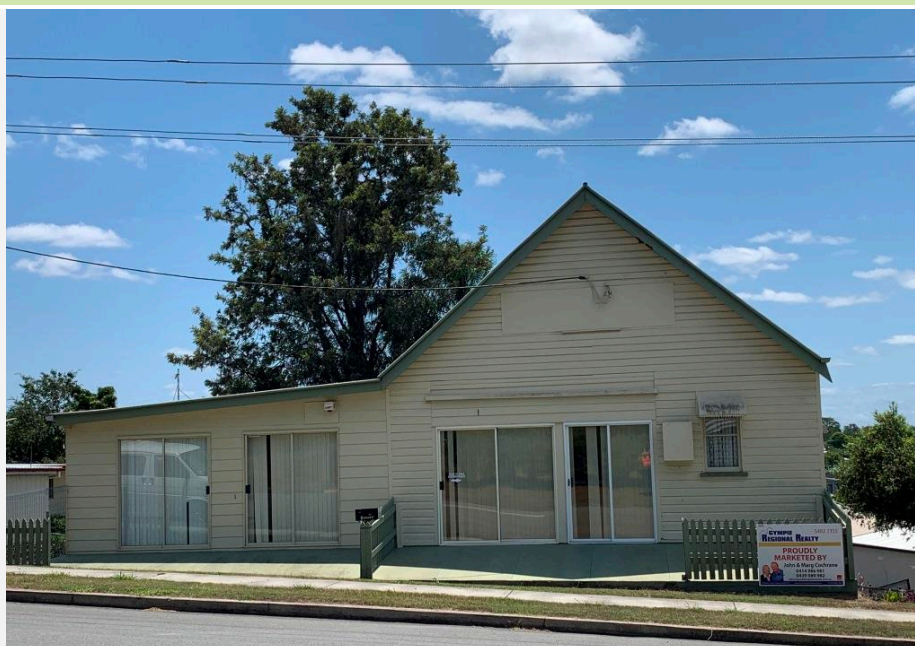
Commercial (former): 8 Graham Street, Gympie, 2019.
