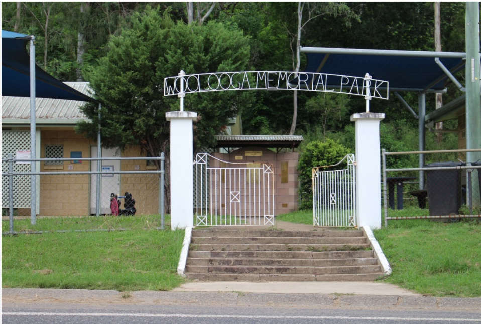
Woolooga Memorial Park and Gates, 2020
