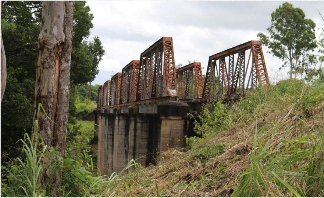
Imbil Railway Bridge, 2020
