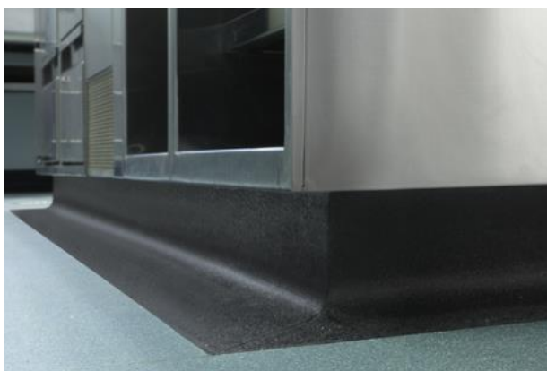
Figure 2: Example of a plinth with coving
