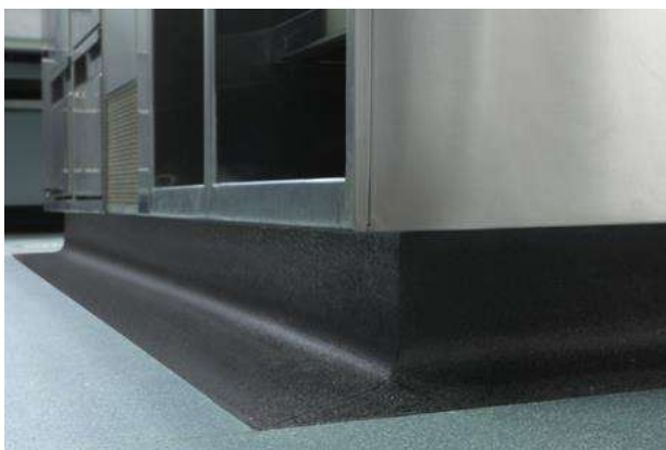
Figure 2: Example of a plinth with coving
