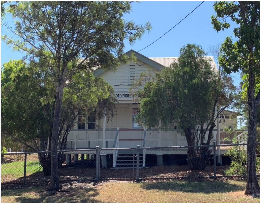
Kilkivan Forestry Office (former), 2020
