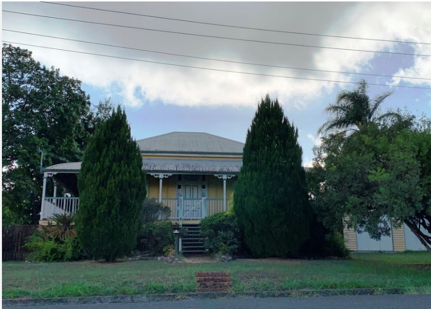
Residence: 12 Watt Street, Gympie, 2019.
