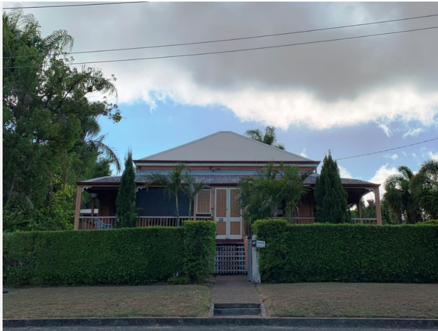
Residence: 14 Watt Street, Gympie, 2019.
