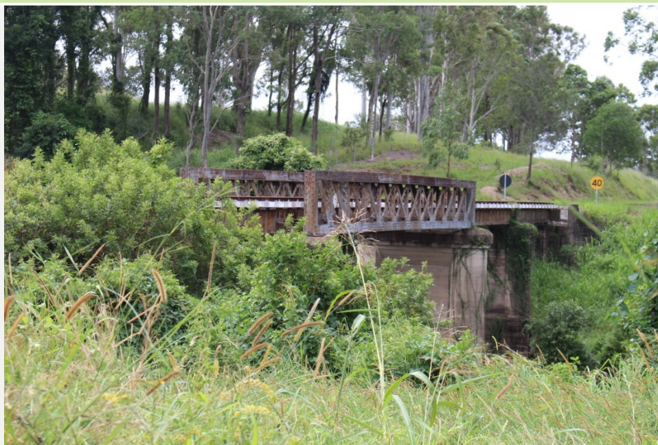
Amamoor Creek Rail Bridge, 2020
