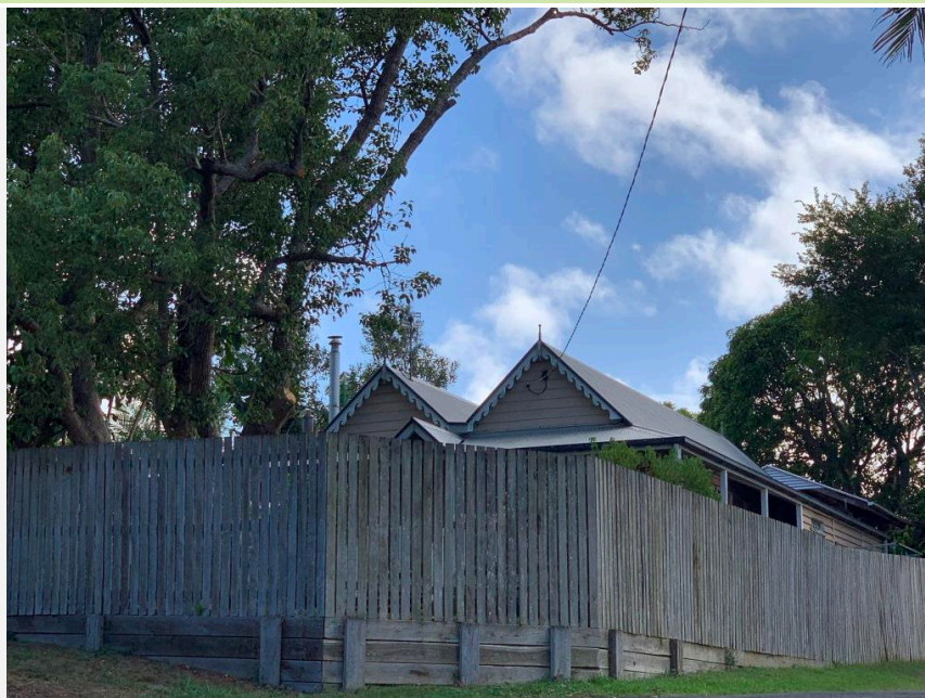
Residence: 18 Watt Street, Gympie, 2019.
