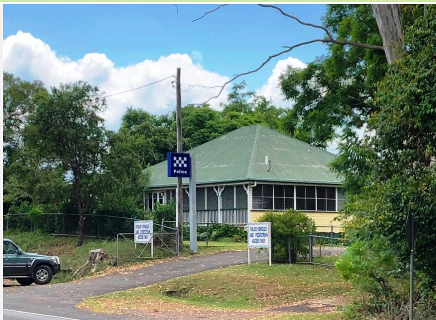
Imbil Police Station, 2019.
