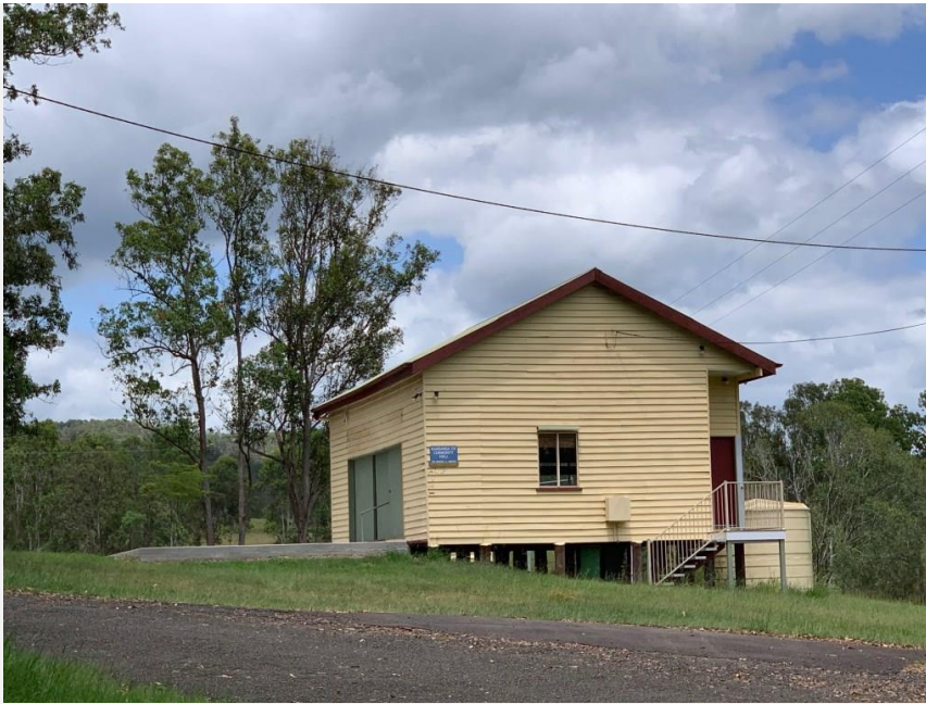
Kandanga Creek Community Hall, 2019.
