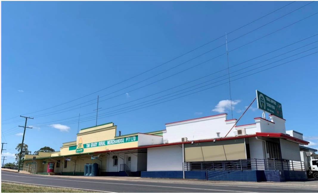
Wide Bay Co-Op Building, 2019.
