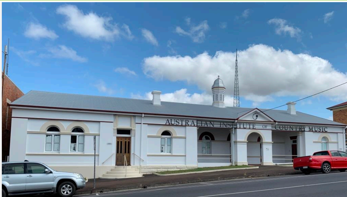
Gympie Court House and Lands Office (former), 2019.
