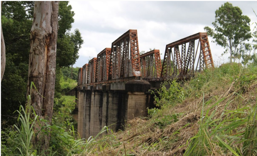
Imbil Railway Bridge, 2020
