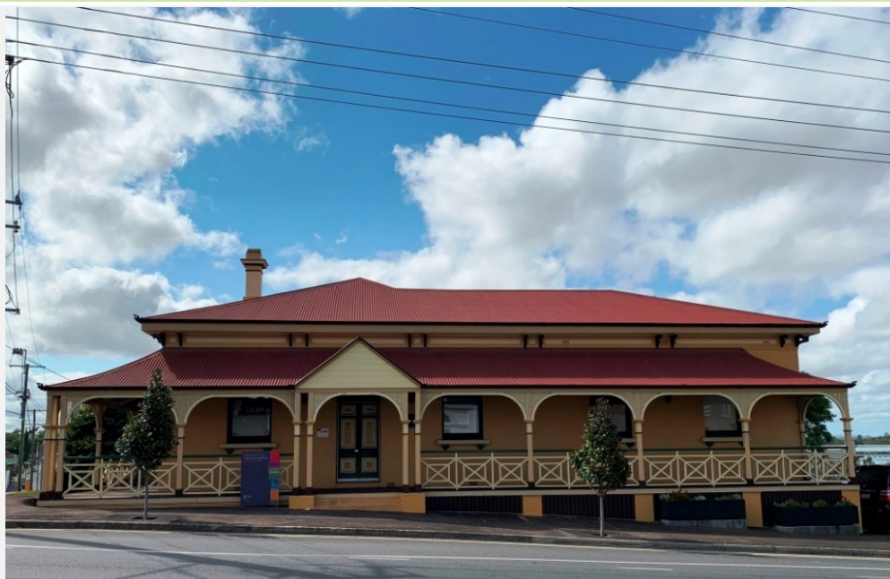
Queensland National Bank (former), 2019.
