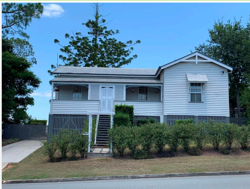
Nashville Police Station (former), 2019.
