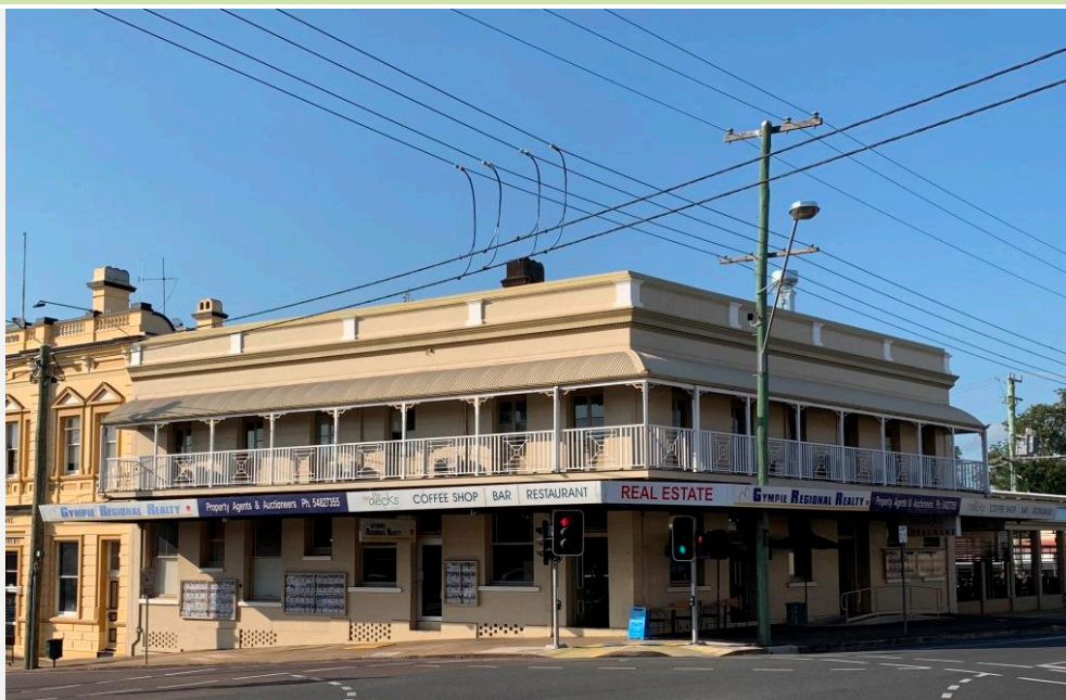
The Commercial Hotel (former), 2019.
