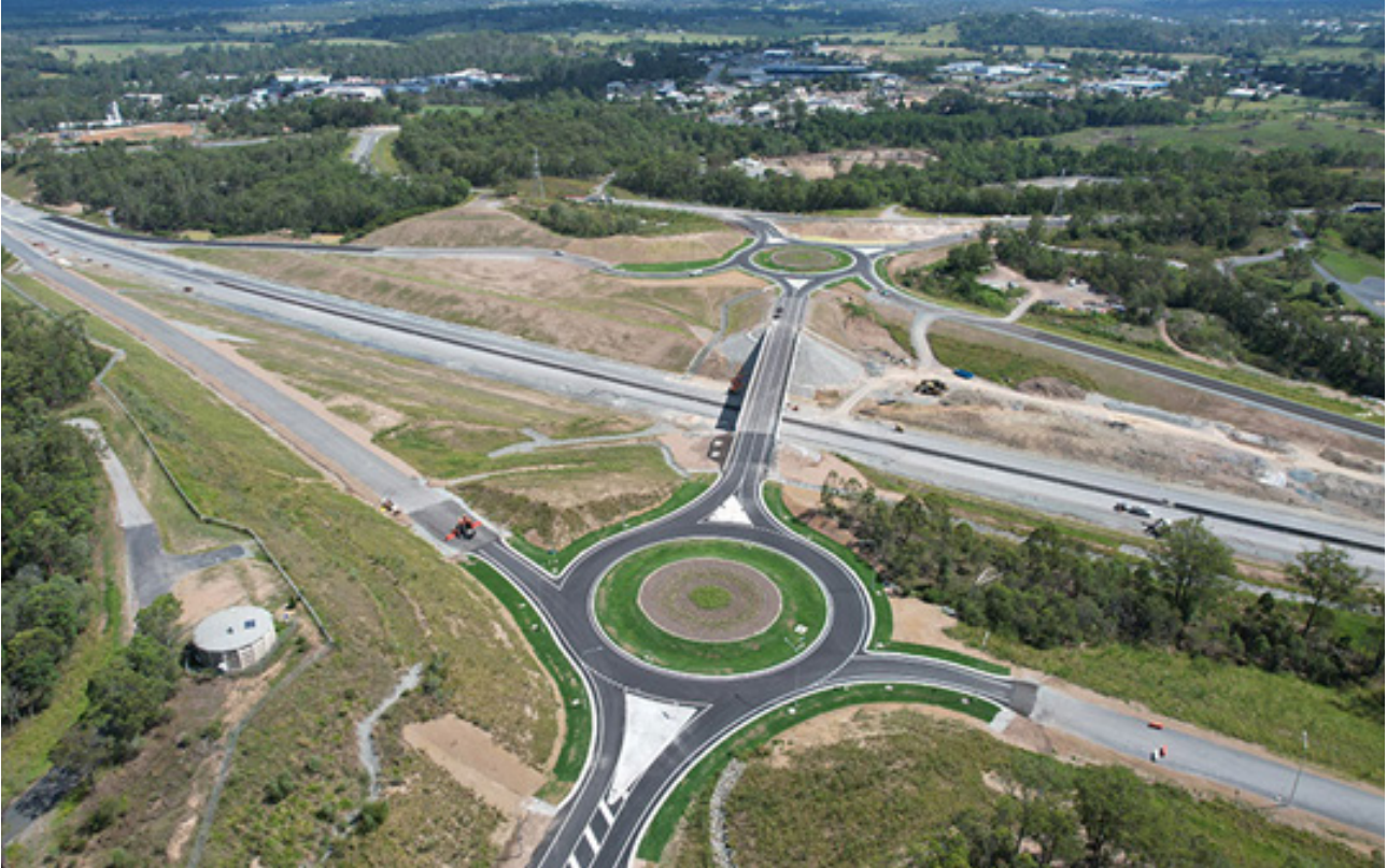
Figure 3: Flood Interchange aerial view of completed work as at December 2022. Image courtesy of tmr.qld.gov.au : Flood Road Interchange design and locality plan
